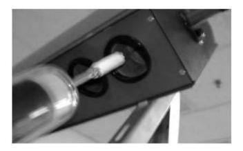
**Step 3:** Slide the tube cap ring over the bottom of the evacuated tube and clip it into place.
